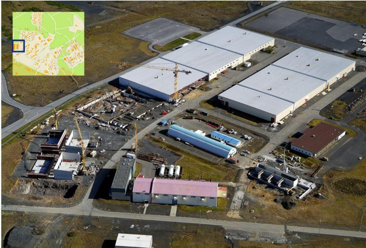
Picture 2. The site (in 2009). Buildings 869 and 868 are the large buildings, 872 is the smaller building on the right (brown roof), 866 is the building in the centre (blue roof) and 864 the building at the bottom (red roof). Other (new) constructions in the picture are constructed by Verne in 2008-9. Source: Socioeconomic impacts of a datacenter in Ásbrú, KPMG Report November 2009 /Verne Holdings ehf.
