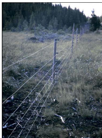
Figure 1. High-tensile electric fence with six wires. (Photo: Norwegian Wildlife Damage Centre, NIBIO Tjøtta/ Inger Hansen).
